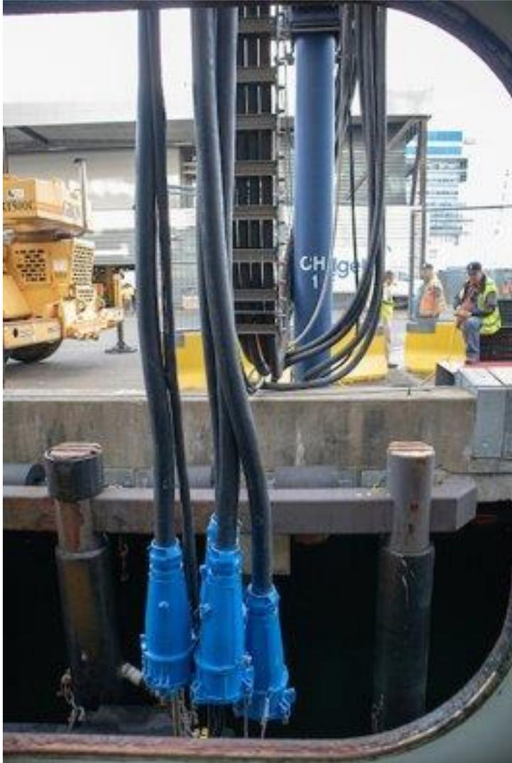
**Scope:** Provide shore power connection for cruise ships while at berth at Pier 66’s Bell Street Pier Cruise Terminal. Power to be provided across Terminal 46 via duct bank and then submarine cable in Elliott bay between terminals. Electrical equipment installed at the south end of Pier 66 will distribute the power to the cruise ship connection.
