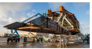
Seven steel fabricators located across the region contributed pre-fabricated components to the pedestrian walkway.
