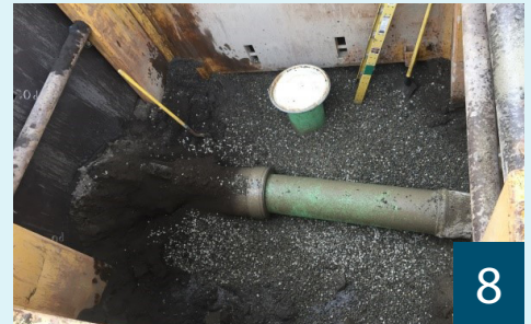
(8) The broken pipe segment is repaired prior to backfill.
