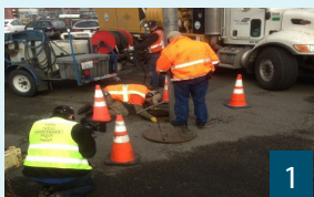
(1) First, the Utility crew sets up their equipment and...
